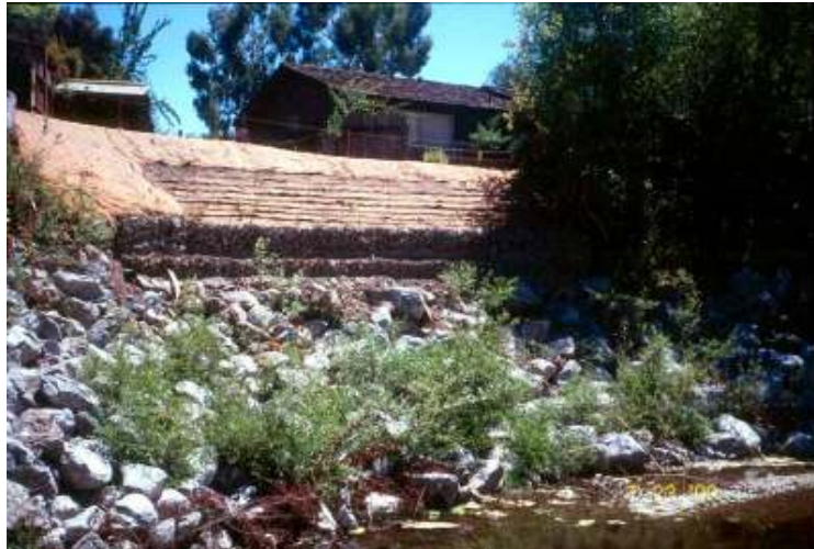
Soil Choked Riprap with plantings
