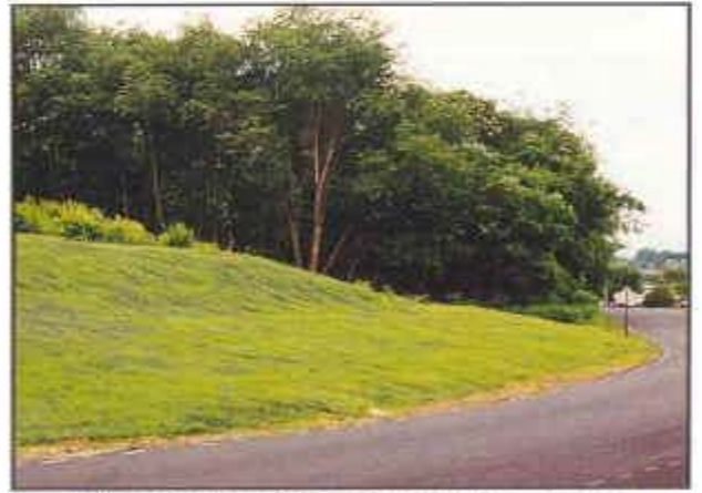
Slope Stabilization—Partially Vegetated TerraGuard™ 45P
