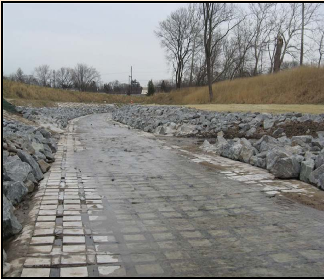
Reconstruction of Rose Valley Creek, looking upstream.
