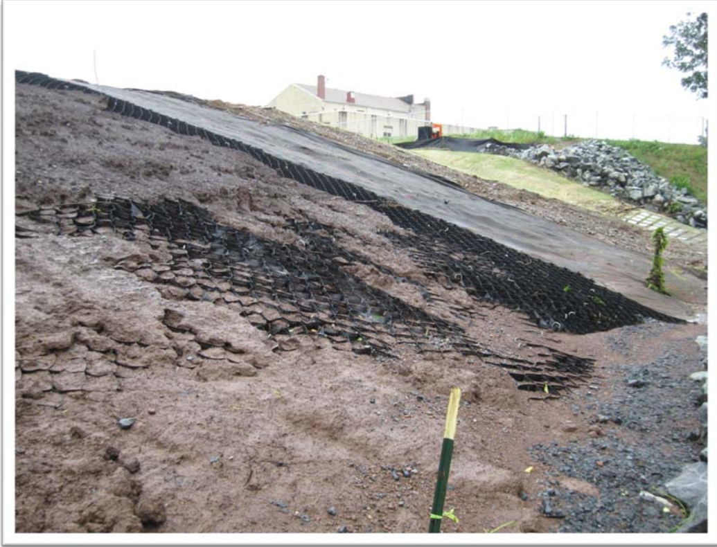
Geocells – Phase V Slope
