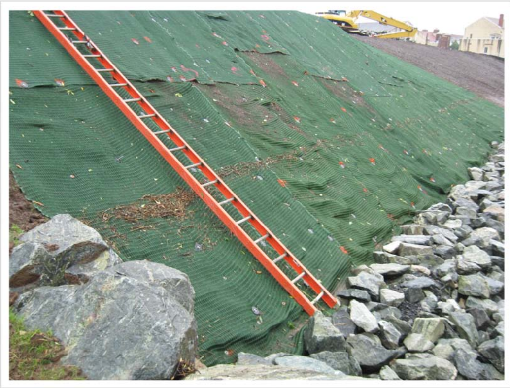
ArmorMax – Phase V Slope
