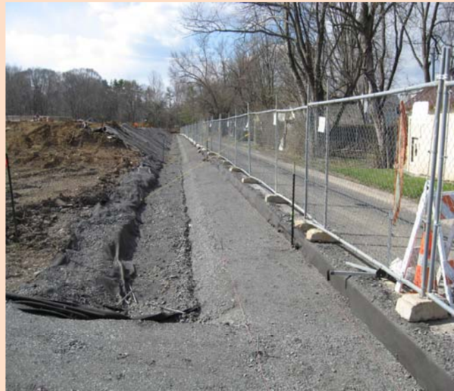
View of the working area along the alleyway by the Rose Valley headwall, facing north.
